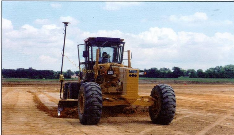
GPS equipped Komatsu Motorgrader cuts grade for building pad.
